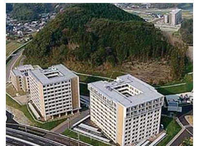
〈 Dormitory 1 and 2, and Ito Harmony House 〉
