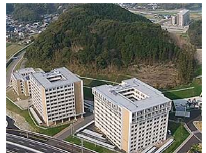
〈 Dormitory 1 and 2, and Ito Harmony House 〉
